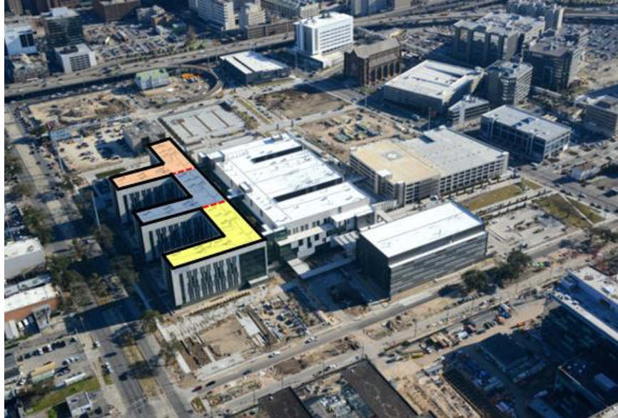
Figure 10 - Inpatient Towers Building Expansion Joints [Courtesy of NBBJ Architects]
